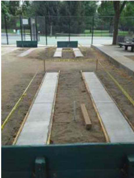
New concrete walkway
